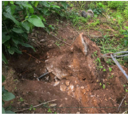
Figure 3. The anchor rope foundation is set on the floating soil.
