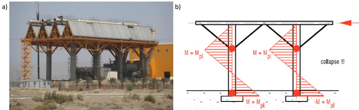
**Figure 1 a.** A concrete ACC structure in Kahnooj, Iran<sup>[1]</sup>, b) formation of plastic flexural-hinges in two ends of concrete columns presumed in strong ground motions<sup>[2]</sup>.
