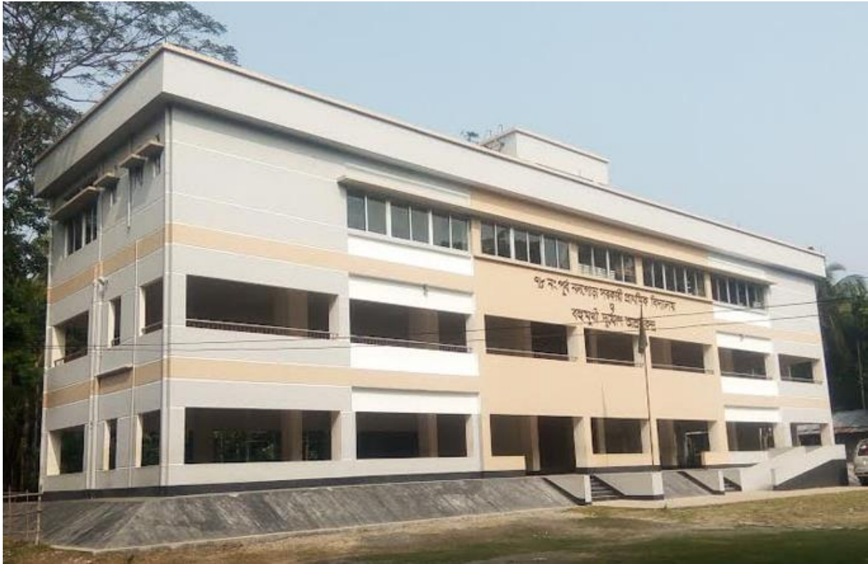
Figure 1 (b). A typical cyclone shelter (school building).
