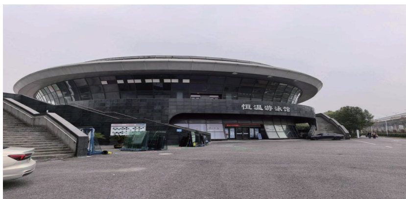
Figure 2. Overall view of the steel structure of a university sports center.
