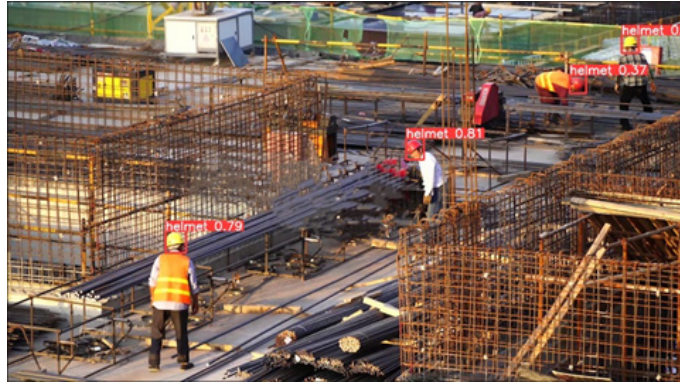
(b) improved YOLOv5 hard hat detection under complex background
