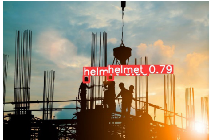
(d) improved YOLOv5 safety helmet detection under uneven lighting
