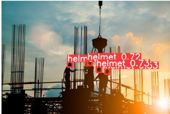
(c) YOLOv5 safety helmet detection under uneven lighting
