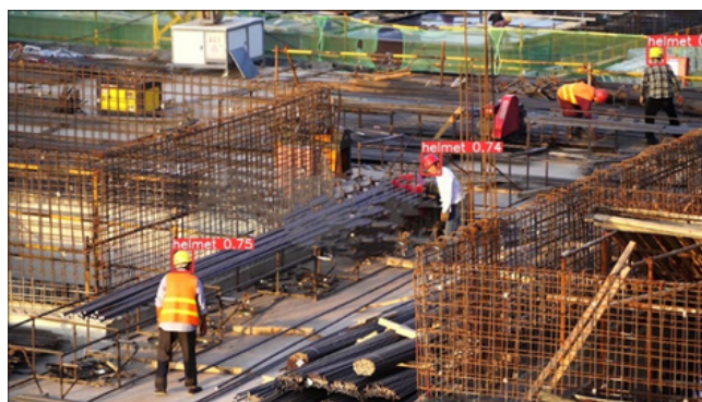
(a) YOLOv5 hard hat detection under complex background
