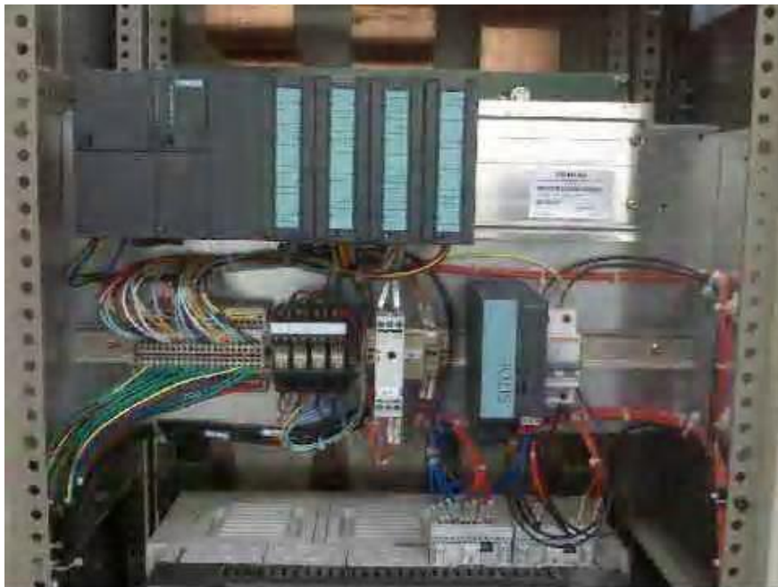
Figure 10. NTC thermistor PLC acquisition hardware diagram.
